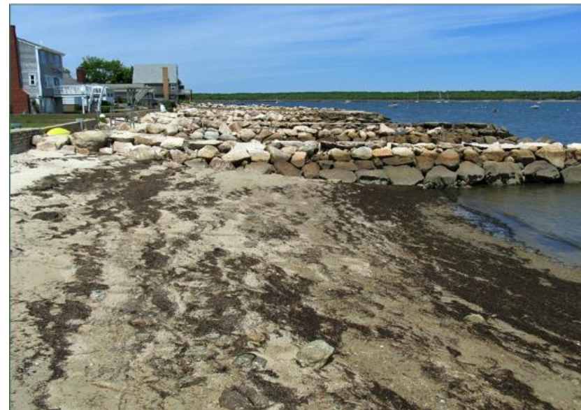
Western shoreline near DV-01b looking northwest at low tide on 31 May 2004.
