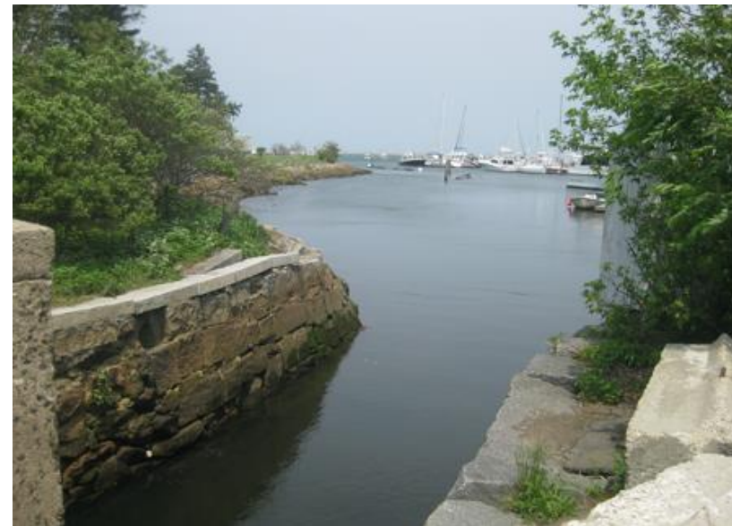
Culvert at Water Street (CB-03)
