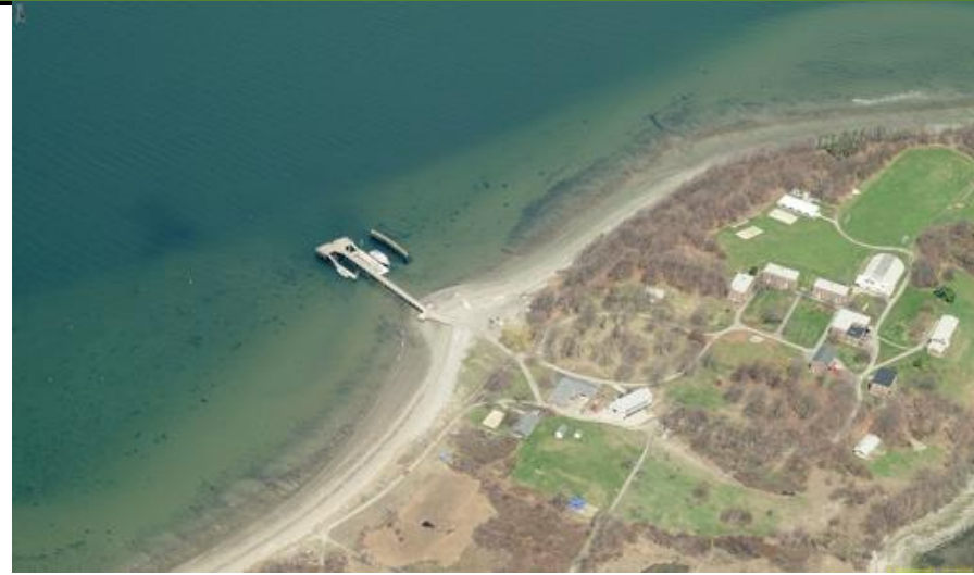
Dock (site access) on NW side of island
