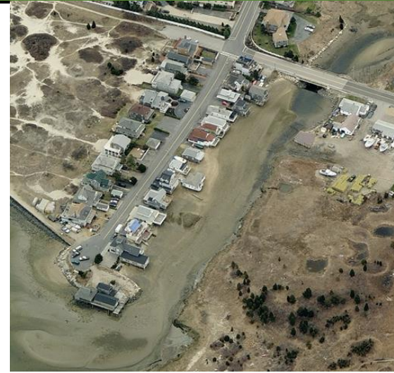
View looking southwest towards the entrance to the marsh behind Beach Street. (EX-02)
