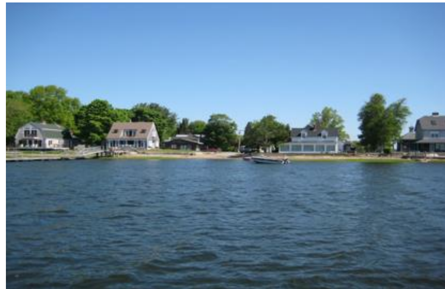
Site of DV-01b and SR at Cottage Rd looking north at high tide on 21 May 2009.
