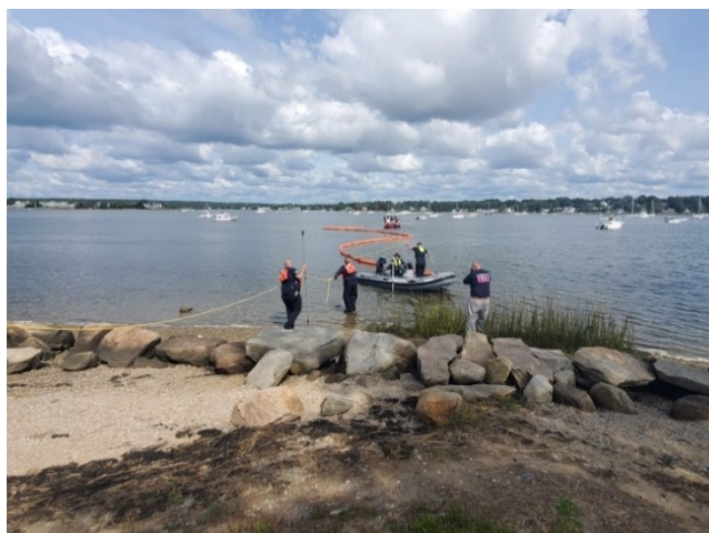
Shoreside crews assist with shore-to-vessel transfer
