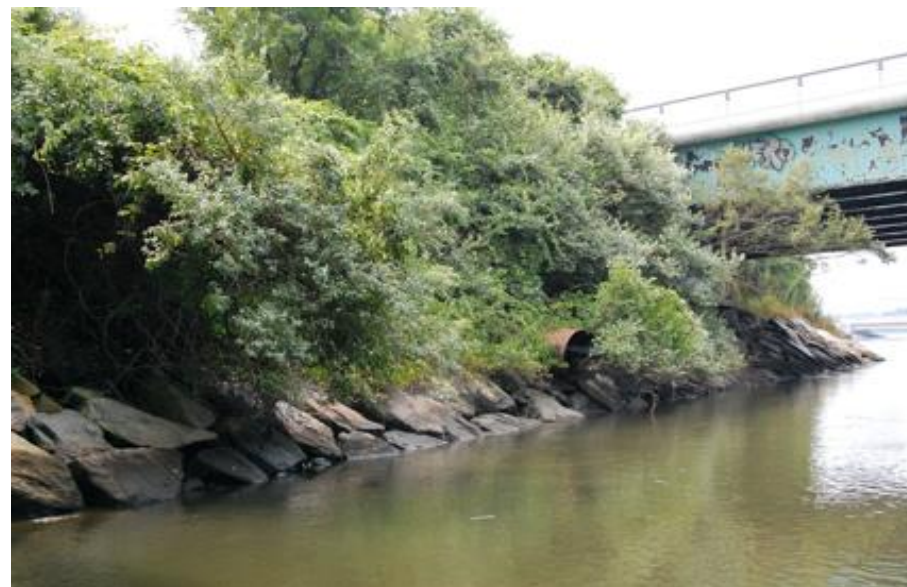
Culvert between I-195 Bridge
