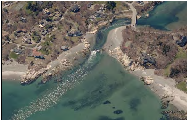
View looking south towards DV-01.
