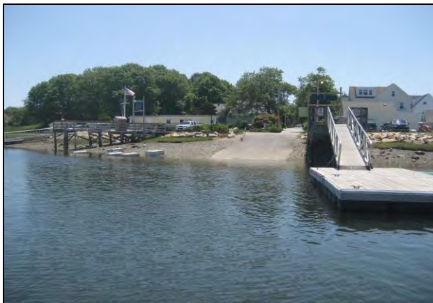
Boat Ramp located at Cohasset Harbor Marina. (GRP SS-02 Inner Cohasset Harbor)
