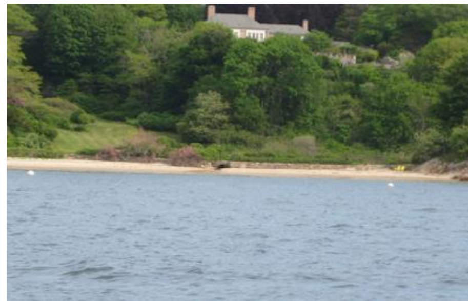
Plum Cove culvert (CB-3b) at mid-tide looking north (02 June 2009 photo)
