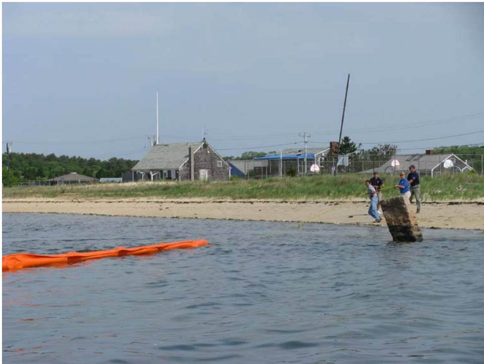
Figure 6. Setting the Shoreline Anchor
