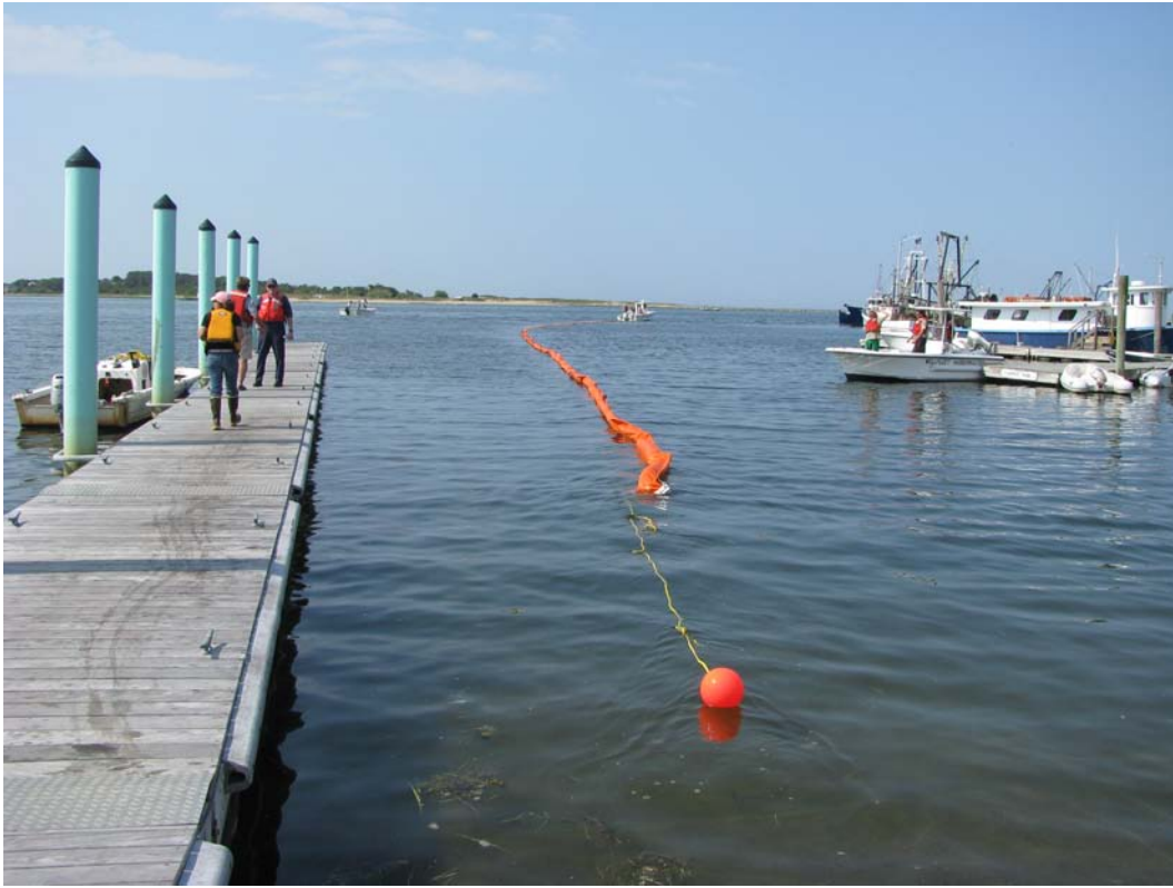
Figure 6. Setting the Shoreline Anchor
