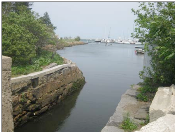
Culvert at Water Street.
