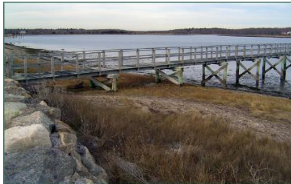
EX-01a western shoreside anchor point looking north at low tide on 10 January 2008.
